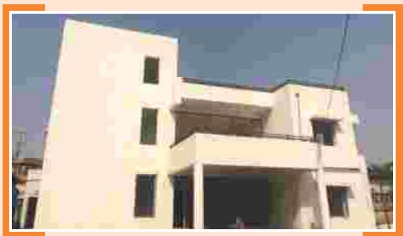
Sainik Rest House Building under construction
